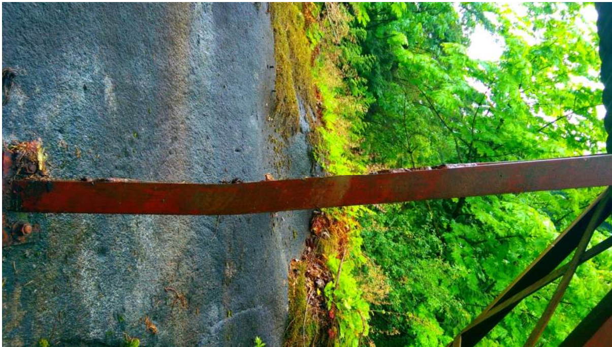
Photograph 8 Bent support leg from falling debris.
