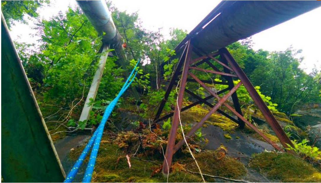
Photograph 3 Typical support bent. North pipe is to the right.
