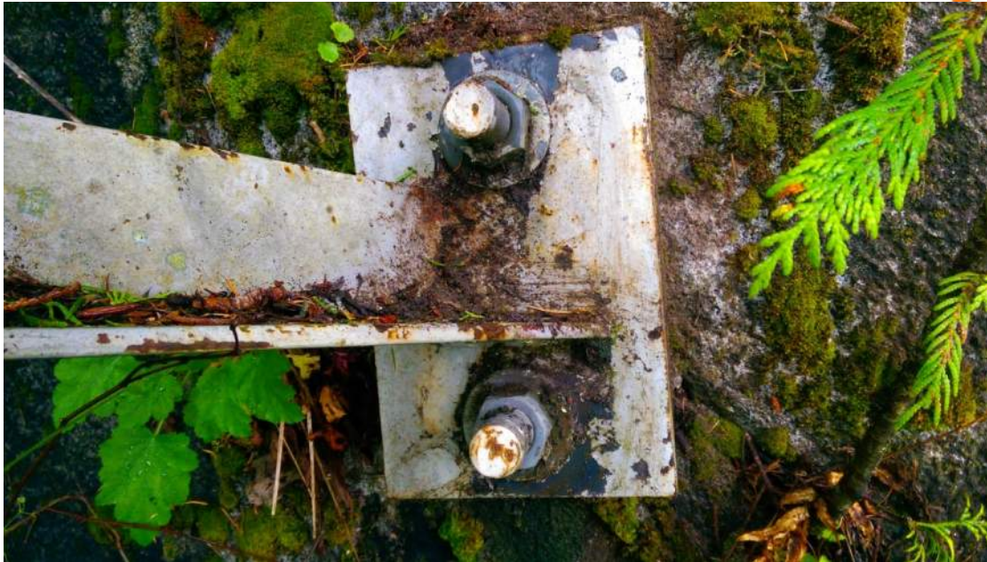
Photograph 5 South pipe support anchor bolts.
