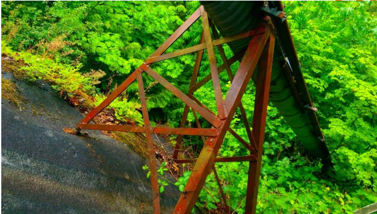
Photograph 7 Typical support frame – north pipe.
