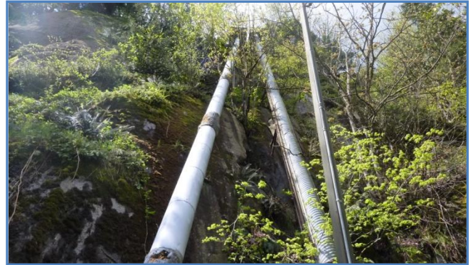
PHOTO 2: Looking up, north pipe is on the right
