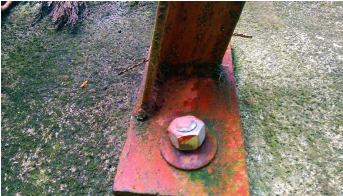
Photograph 4 North bent baseplate and anchor bolts.
