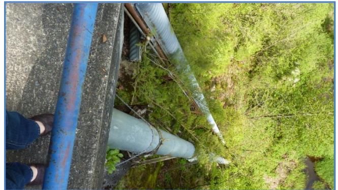
PHOTO 4: Looking down, north pipe is on the left
