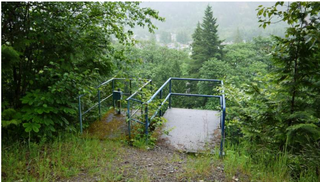
Photograph 2 Top concrete abutments. Concrete work is in average condition.
