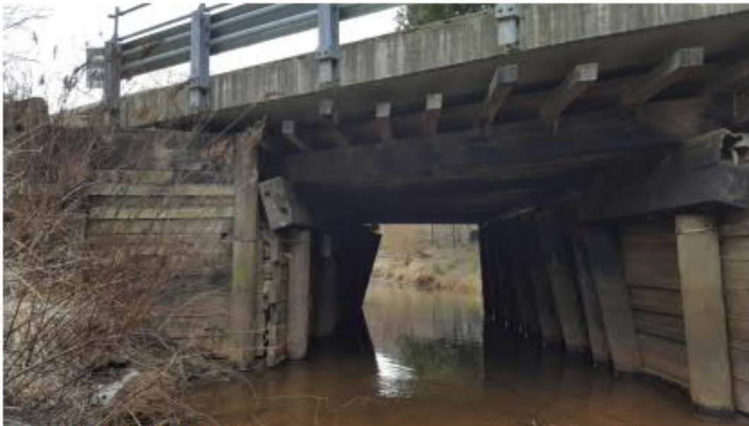
Photo 2: Side view of bridge
