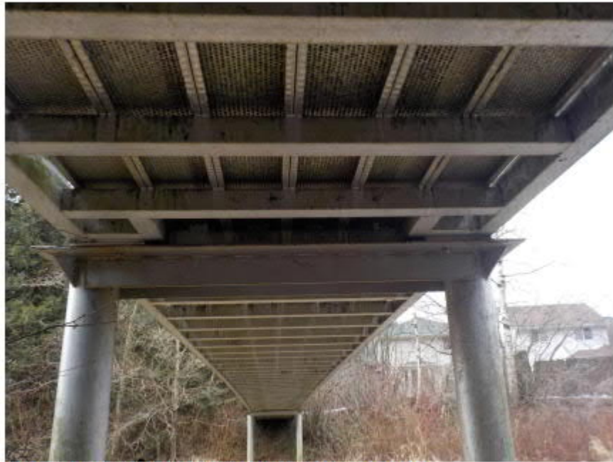
Photo 3: View of underside of bridge and pier support
