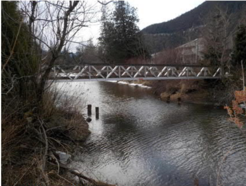
Photo 1: Side view of bridge
