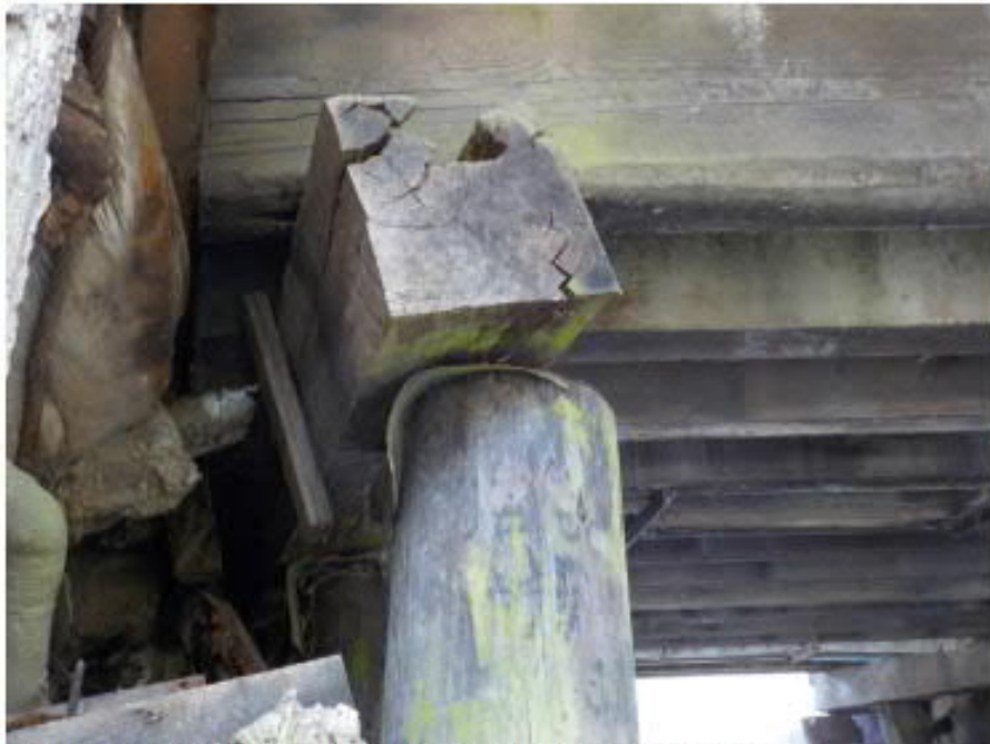
Photo 6: Cap beam and timber pile connection at south abutment
