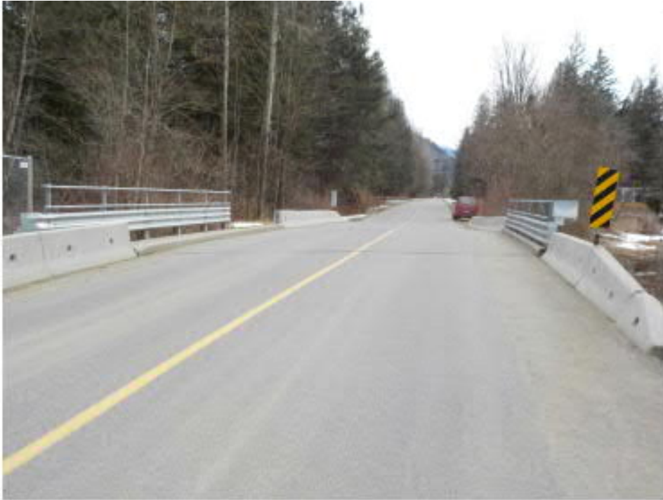
Photo 1: Approach view of bridge
