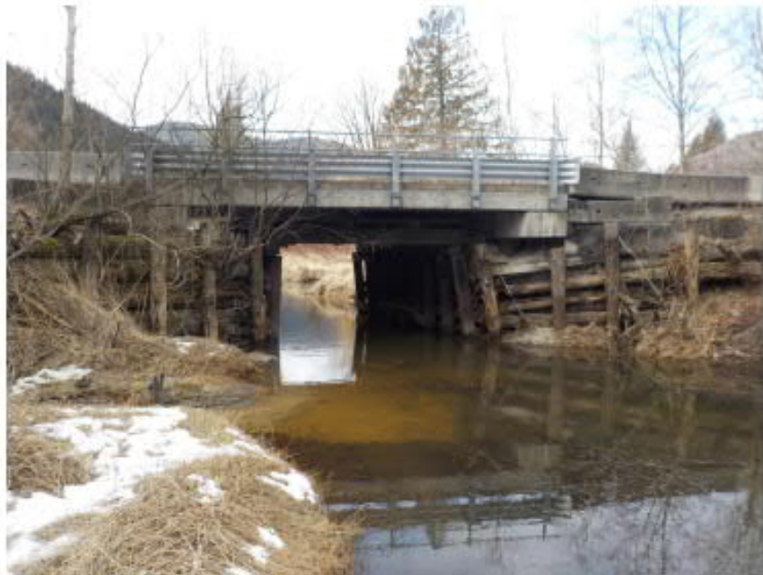
Photo 2: Side view of bridge
