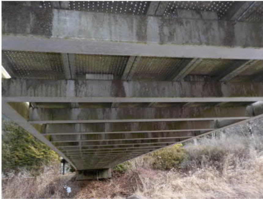
Photo 3: View of underside of bridge
