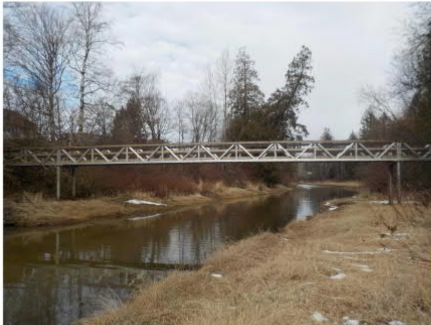
Photo 1: Side view of bridge
