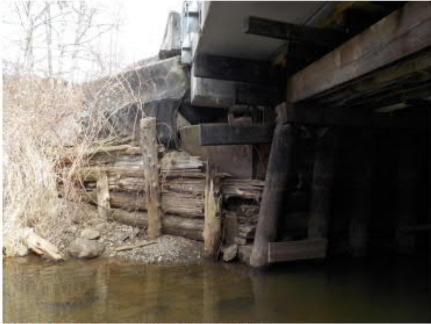
Photo 5: Timber piles and ballast logs at wingwall
