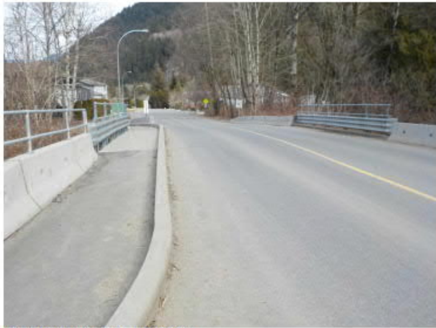
Photo 1: Approach view of bridge
