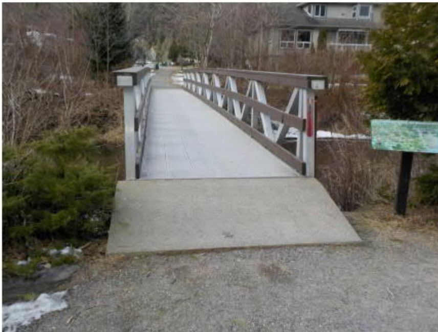
Photo 2: Approach view of bridge
