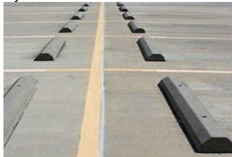
Sample only of a Concrete Barrier at the end of the stall
