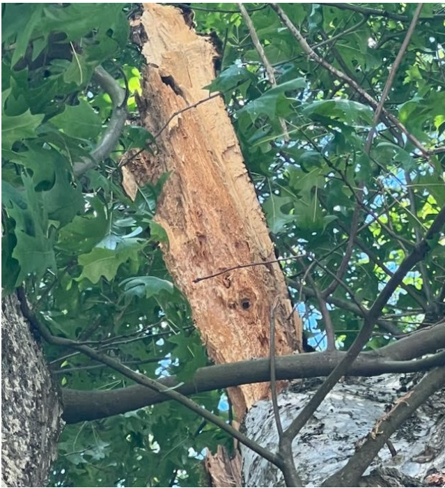
Fig.5 – Recent branch failure, tree 407.
