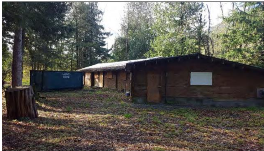
Photo of the derelict building 410 Echo Avenue
