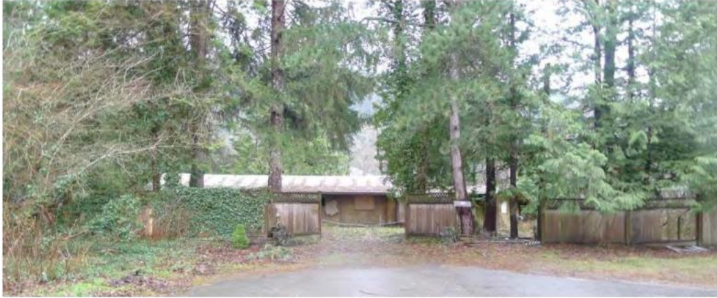
Photo of the derelict building 410 Echo Avenue
