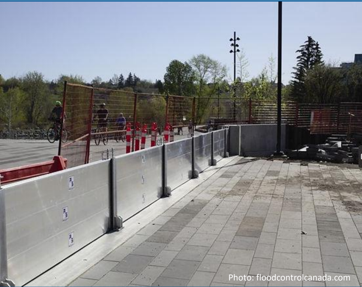
Deployable flood wall installed during flood events
