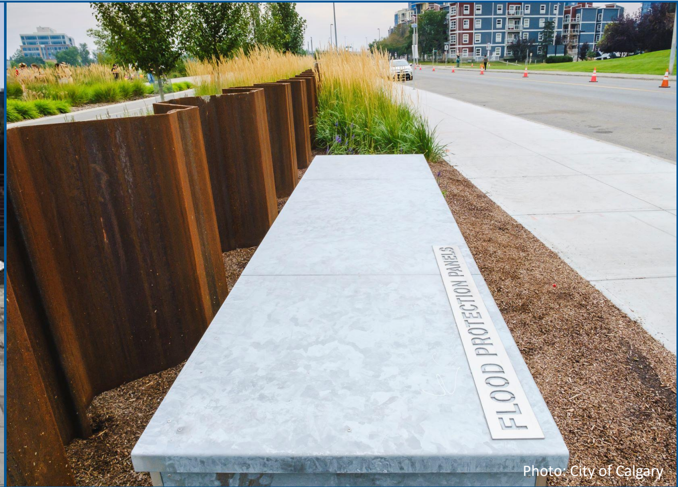
Deployable flood wall stored in boxes adjacent to openings
